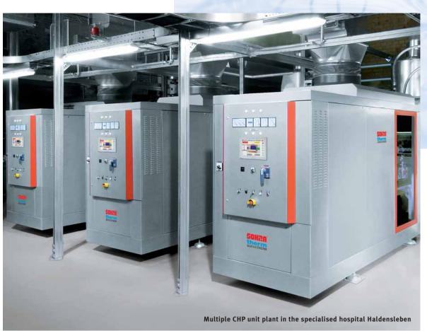
The combination of multiple CHP units allows an energy supply in the power range of Megawatts.
